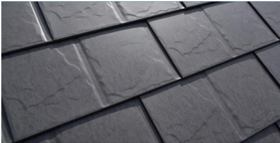
Figure 1 – Typical Interlocking Metal Shingle Roof
