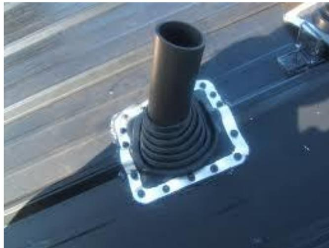
Figure 4 – A Square Base Flashing is shown on a roof vent pipe fastened to the metal roof with sealant and small sheet metal screws.
