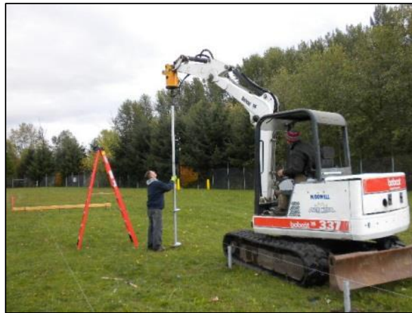
Figure 1 – Auger being driven at Groundwater site with Bobcat 337
